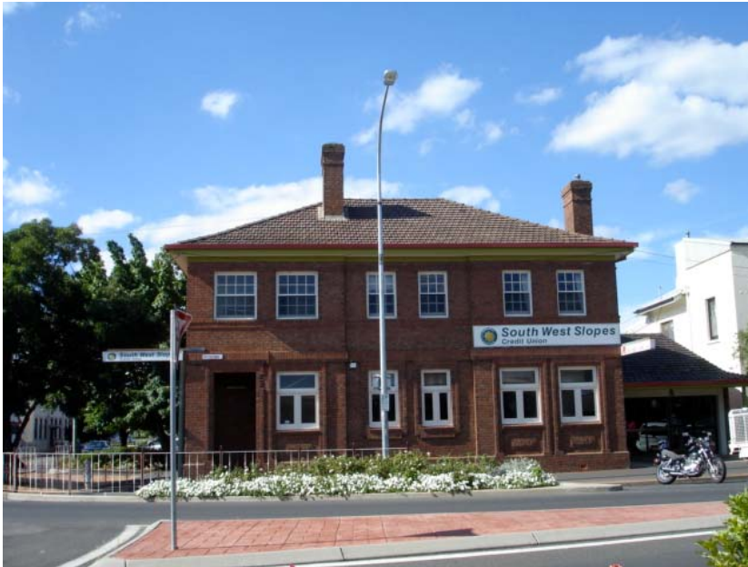
South West Slopes Credit Union after repainting.
